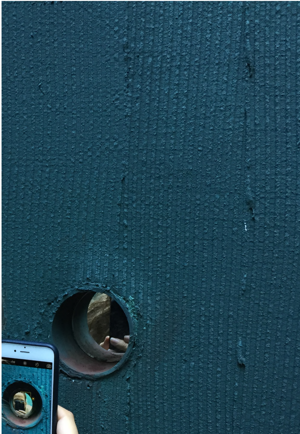
photograph taken at Pezo von Ellrichshausen's Vara Pavilion at the Venice Biennale, July 2016
